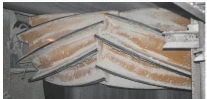
Figure 7 – Herringbone wing in underground quarry.
