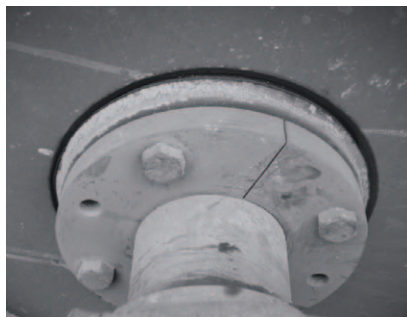
Figure 2. A common welded steel pulley failure.
