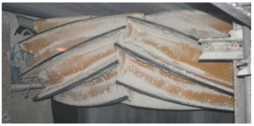
Figure 7 – Herringbone wing in underground quarry.
